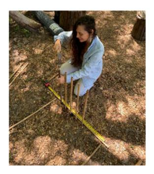
Step 7- We lay another piece of bamboo to measure the length from the set bamboo stakes to
