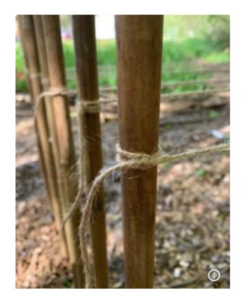
Step 9- Create the tension bar and tie the jute in the middle spaces left to the tension bar.
