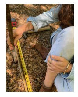
Step 6- Working out drive all your holes and then stake them there are 9 total entering the ground so four on each side of the center. Divide the center 30inches by eight to get your pole placements.
